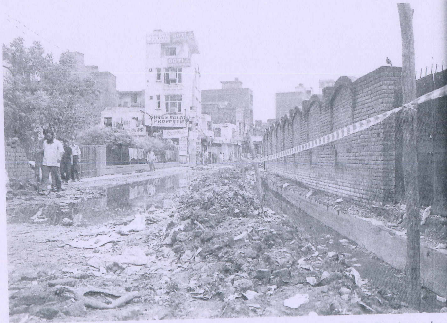
A typical monsoon scenario of a road, which is one of the main roads leading into a low income residential colony.
